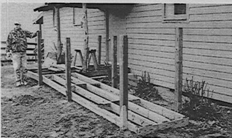
Ralph Jurgens inspects posts installed for access ramp.
